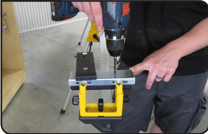
PRE-DRILL HOLES FOR ADAPTER BLOCK
